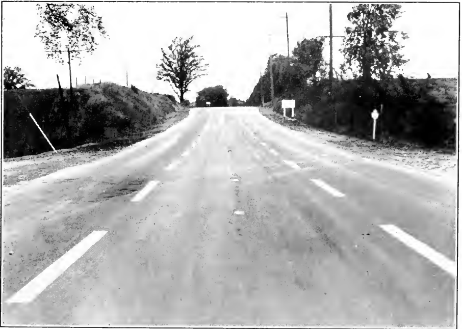
Asphalt Pavement, Highway No. 11, Showing Widened Pavement.
